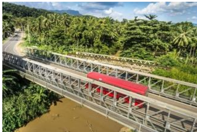
Figure 22: Modular bridge deck panels with pedestrian way for heavy-duty highways bridges (Mabey, 2016)
