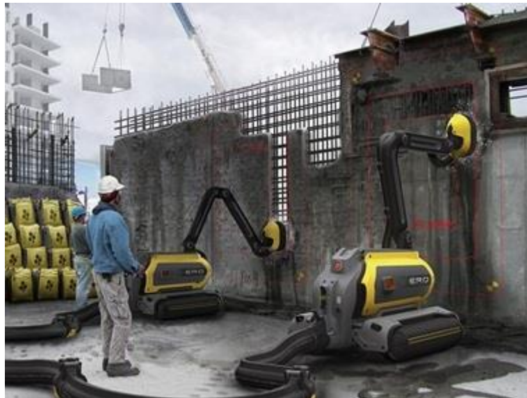
Figure 17: A semi-autonomous concrete recycling robot (Haciomeroglu, 2012)
