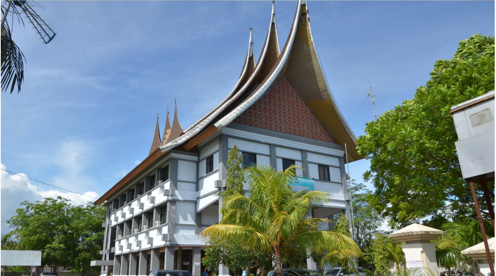
BUNG HATTA UNIVERSITY BUILDING (Jalan Khatib Suleman, Padang)
