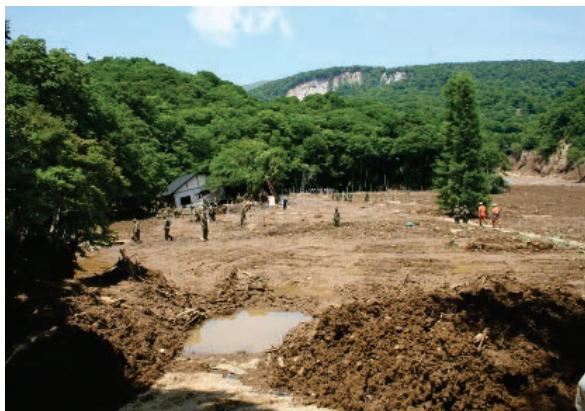
Photo 1. Mudflow type slope failures of 2003 & 2008 Earthquake in JAPAN
