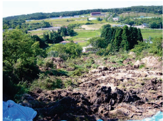
Photo 1. Mudflow type slope failures of 2003 & 2008 Earthquake in JAPAN
