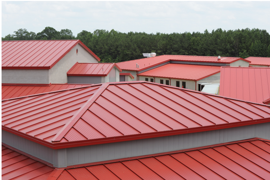
Figure 4.27. Application of roof sandwich panels
