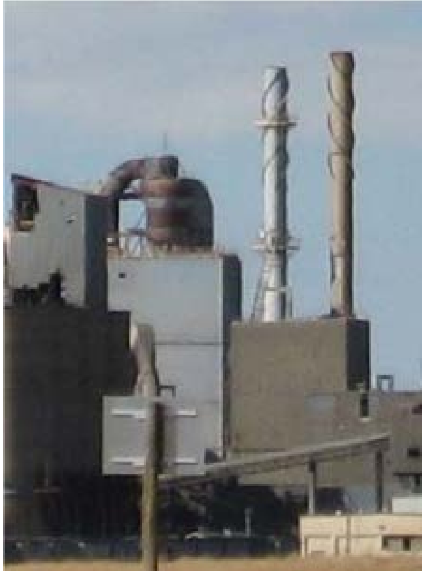
Figure 3.6 Stacks in Laramie, WY retrofitted with helical strakes [3]
