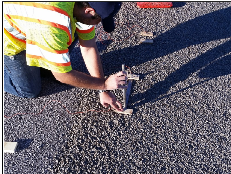
Figure 4.24: Tapping steel rod probes.
