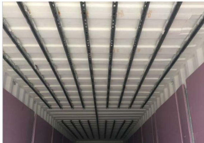
Figure 3.4. Strut channel pieces welded to ceiling of shipping container.
