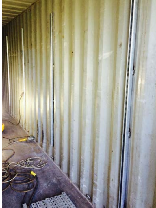
Figure 3.3. Strut channel pieces welded to walls of shipping container.
