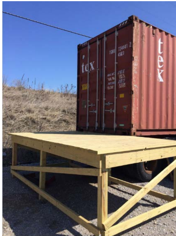
Figure 3.1. Existing doors of the shipping container will serve as the entrance.
