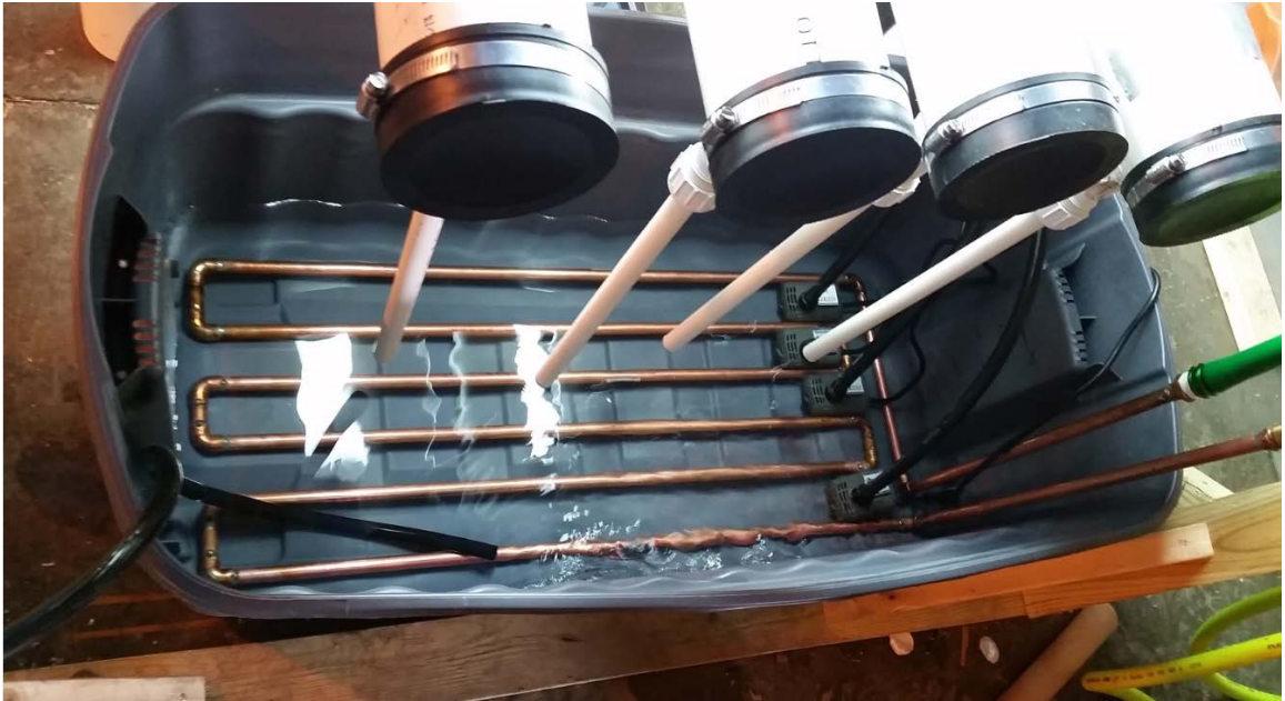
Figure 5.2. Cooling coil placed in reservoir to lower water temperature.
