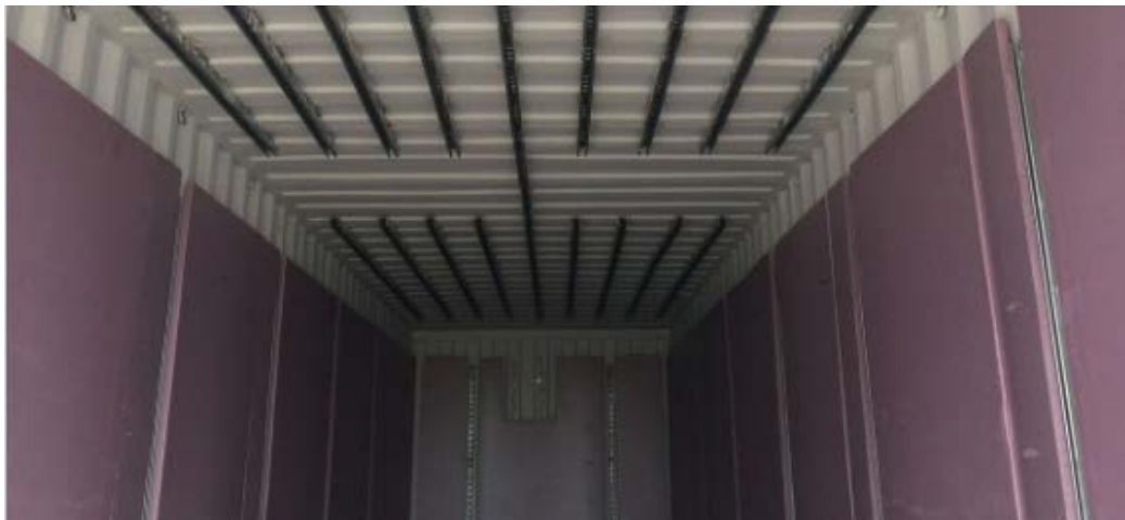
Figure 3.15. Insulation on all walls of container.
