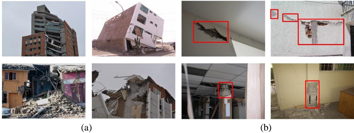
Figure 5.4 Samples of ground truth (labeled) images: (a) collapse and (b) spalling.
