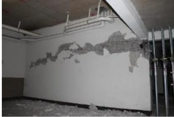
Figure 4.1 Sample image of reinforced concrete shear wall damage in the 2010 Chile earthquake (Moehle et al., 2011; Telleen et al., 2012).
