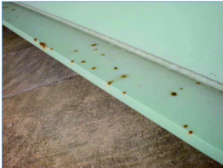
Figure 4.4: Portion of a steel girder candidate for spot painting (Myers et al., 2010)
