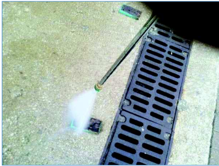
Figure 5.12: Power washing steel coupons
