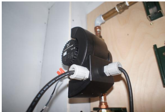
Figure 3-11. Water pump.
