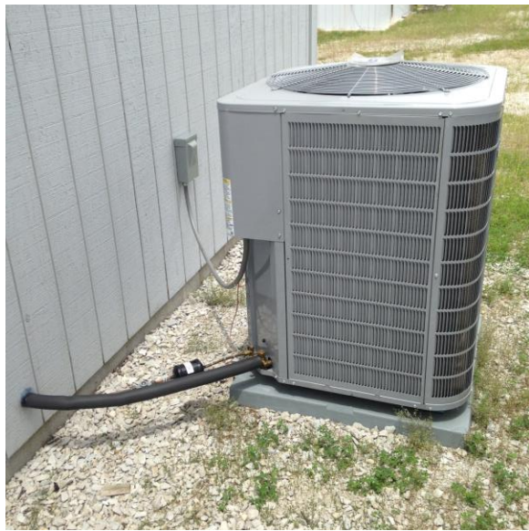
Figure 3-4. Vapor-compression refrigeration unit.
