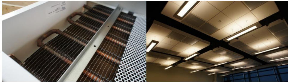
Figure 1-2. Passive chilled beam and perforated panel.
