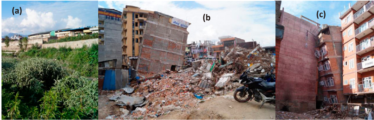
Fig. 13. (a) Building on soft lake deposits with Kathmandu (b) and (c) examples of collapsed buildings within Kathmandu in vicinity to Fig. 13(a).
