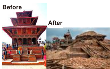
Fig. 16. Harishankar temple before and after the earthquake.
