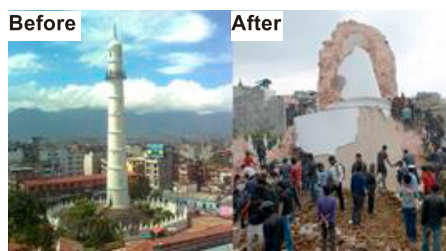
Fig. 14. State of damage of Dharahara tower.
