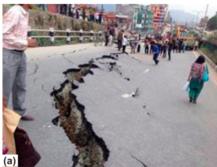
Fig. 8. Slope failure and subsidence (Bhaktapur side) (a) subsidence of the access road and (b) tilted apartment building.
