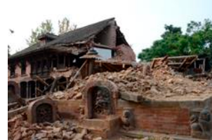
Fig. 23. One of the collapsed temples in Changu Narayan.
