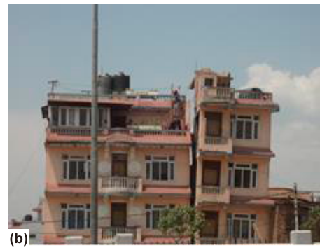
Fig. 8. Slope failure and subsidence (Bhaktapur side) (a) subsidence of the access road and (b) tilted apartment building.
