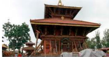
Fig. 22. Two-tiered pagoda after the earthquake protected by scaffolding.
