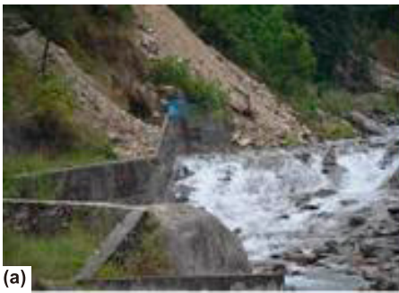
Fig. 36. Earthquake induced landslide (a) landslide in the upstream of intake and (b) landslide in the right bank of headworks.
