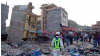
Fig. 29. A typical case of damage to comparatively short buildings.
