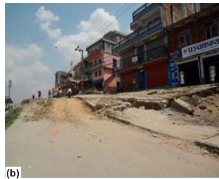
Fig. 7. Slope failure and subsidence (Bhaktapur side) (a) main road and (b) access road.
