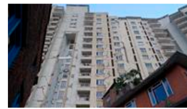
Fig. 30. A typical case of damage to comparatively short buildings.
