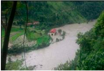
Fig. 33. Submerged power station (Courtesy: Sanima Hydropower Ltd., Kathmandu).
