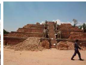
Fig. 18. Vatsala Durga temple after the earthquake.
