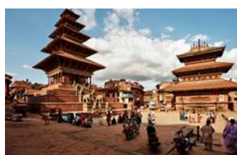
Fig. 17. Vatsala Durga temple before the earthquake.
