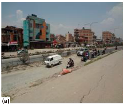
Fig. 7. Slope failure and subsidence (Bhaktapur side) (a) main road and (b) access road.
