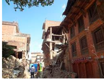
Fig. 27. View of the spot in Fig. 15 after the earthquake.
