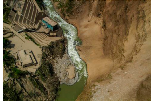
Fig. 6. Partially dammed Bhote Koshi River upstream from the Upper Bhote Koshi Powerhouse. Note extensive dust and talus on the right bank of the river.
