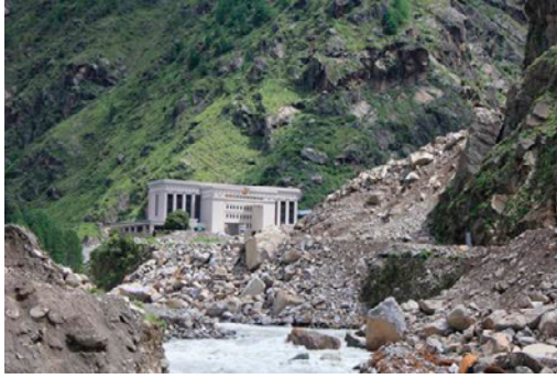
Fig. 3. Partially dammed Bhote Koshi River at the Rasuwa Gadhi check point in the Rasuwa District.
