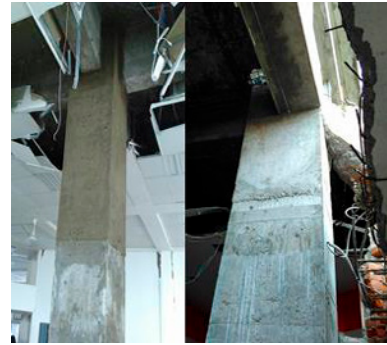
Fig. 16. Concrete jacking at Beam-Column joint, Kathmandu University Central, Dhulikhel.
