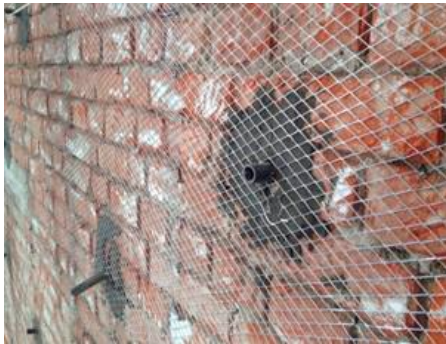
Fig. 17. Retrofitting of wall by net plastering and grouting.
