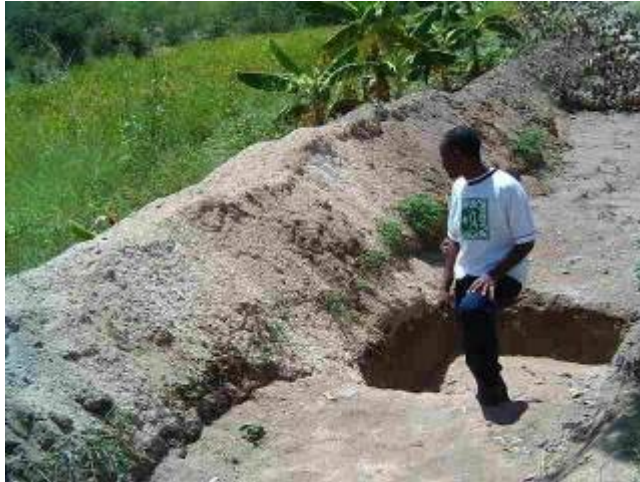
Figure 4.4 A dead (zero-gradient) level contour with water harvesting pits at Sunrise Environmental Action Group in Mutare District.
