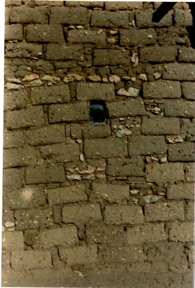
Illus.46. A viewing-hole made by inserting a small piece of glass into an opening in the wall during the construction process
