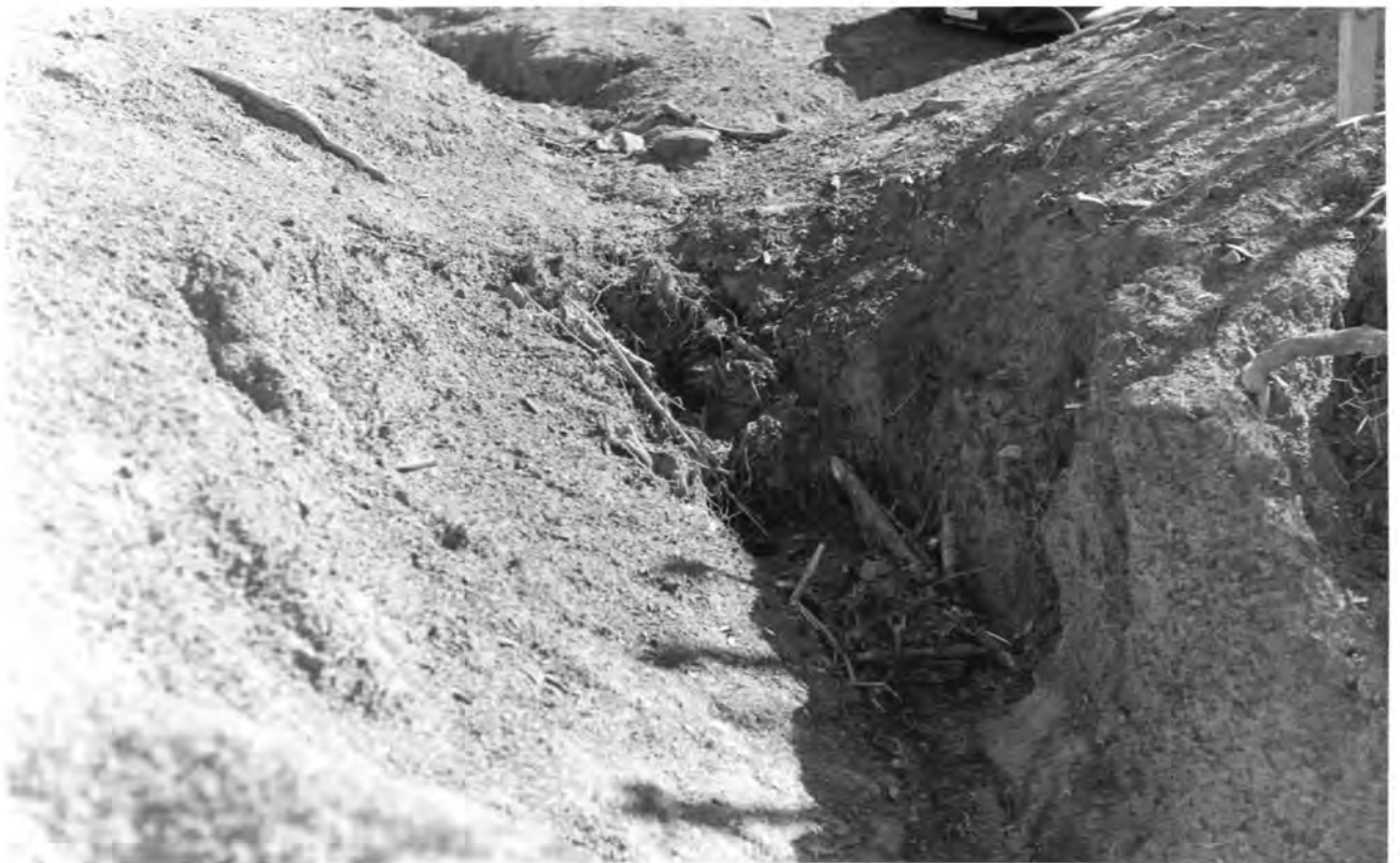
Plate 7.2b. The erosion pin registers erosion in the rill.
