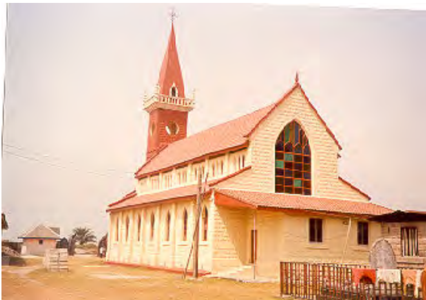
Plate 6.6 Front and rear views of renovated Qua Iboe Church and Tower at Upenekang-Ibeno by Exxon-Mobil, Ibeno LGA
