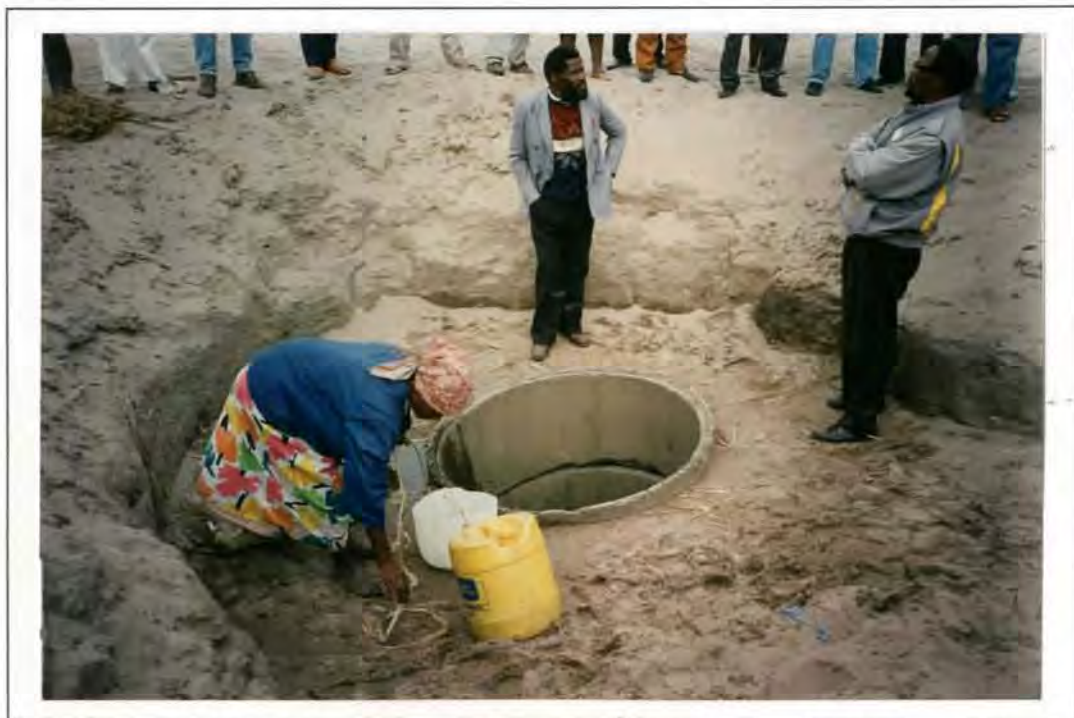
Plate 9. An unprotected hand-dug well being utilised by a local community on the Zululand coastal plain. Note the lifting device is a plastic container with a roughly made palm leaf rope.
