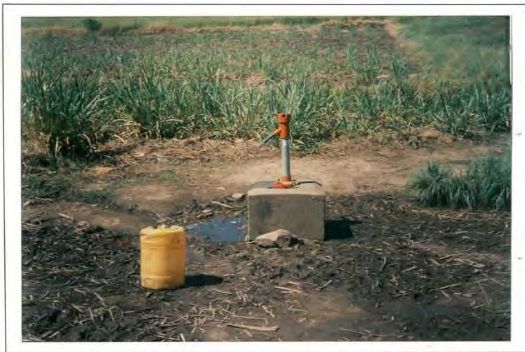
Plate 2. Ponding of spilt groundwater around the bore head is a common problem in KwaZulu-Natal, increasing the probability of contaminated groundwater.
