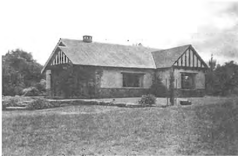
The stone and timber house Brettell built in Nyanga Reproduced with permission of Rosemary Brettell.
