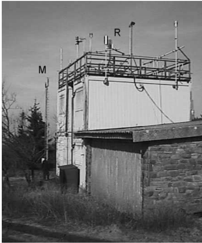
Figure 8.4: Photo of the container tower on Kleiner Feldberg used for measurements after 1996. The photo is taken from the south. The CA intake is marked by the letter ‘R’ and the mast used by the DWD by ‘M’. Photo courtesy of Dr R. Kurtenbach, Wuppertal University.
