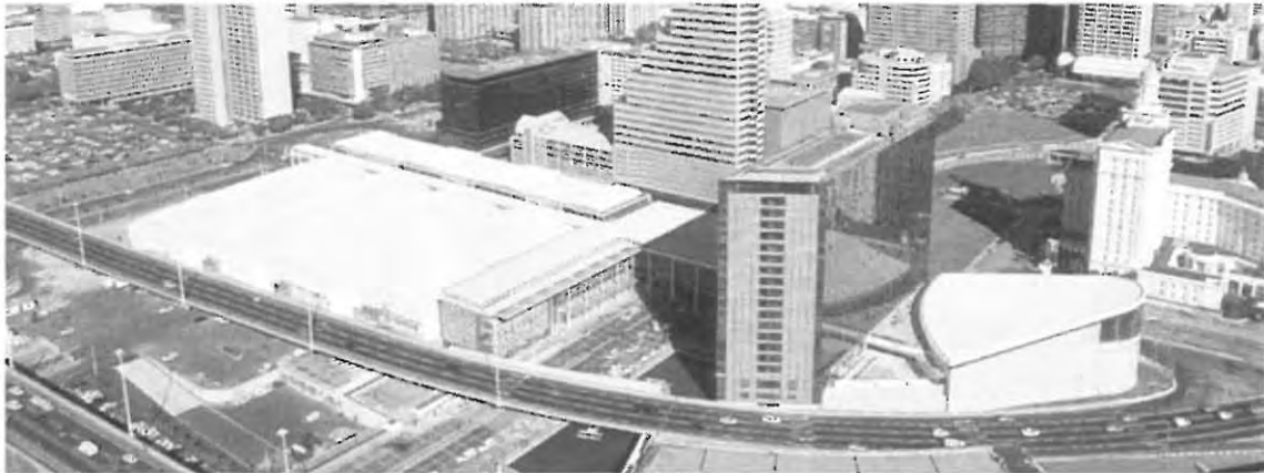
Plate 5.6 Exterior view of the Cape Town International Convention Centre
