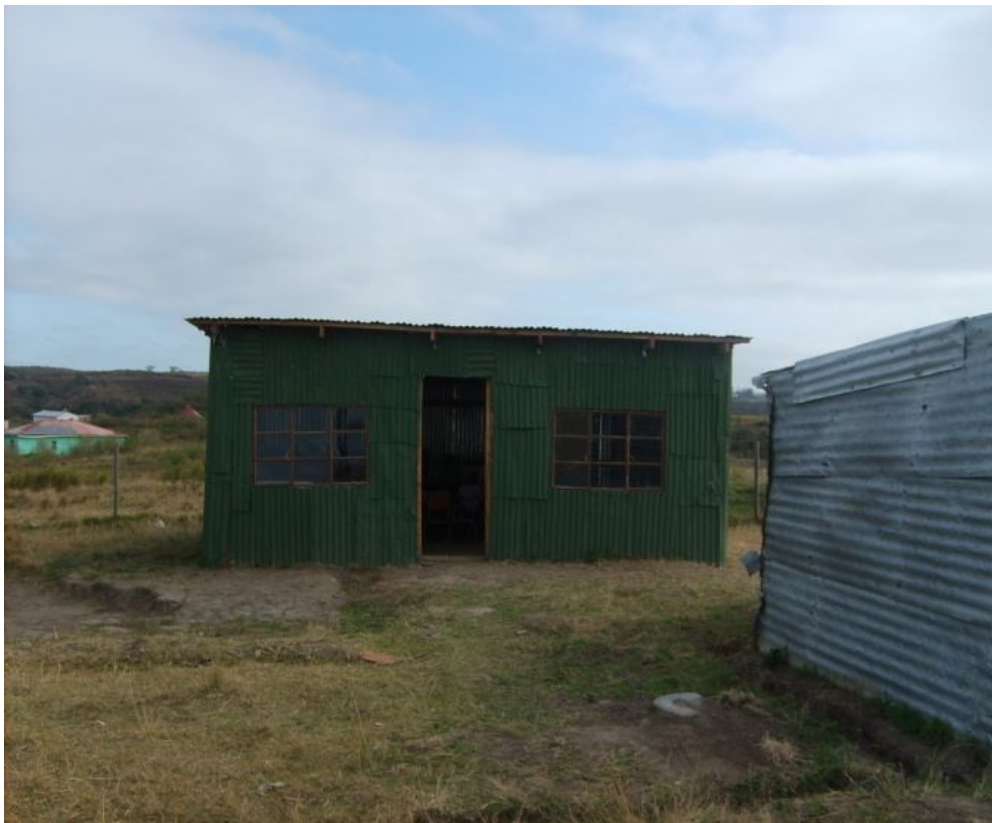
Figure 2:3: Entubeni JSS grade one classroom
