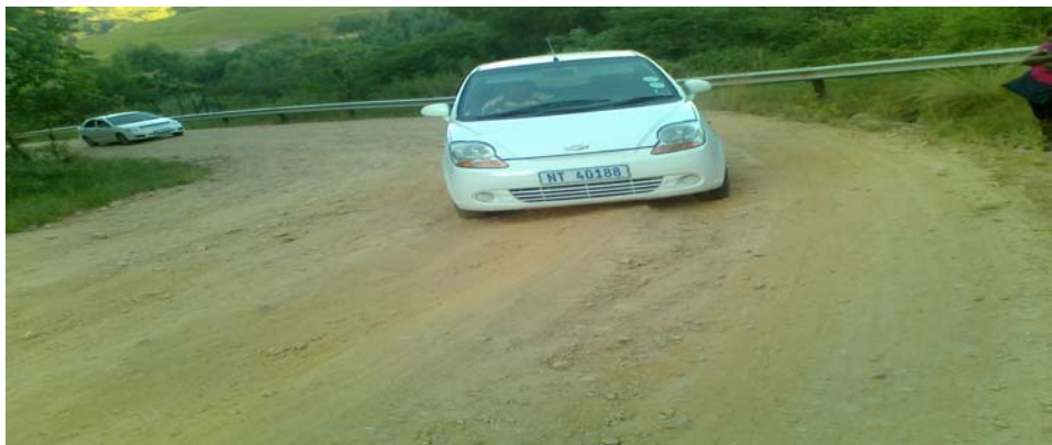
Picture 6.7 Bad condition of roads in rural areas
