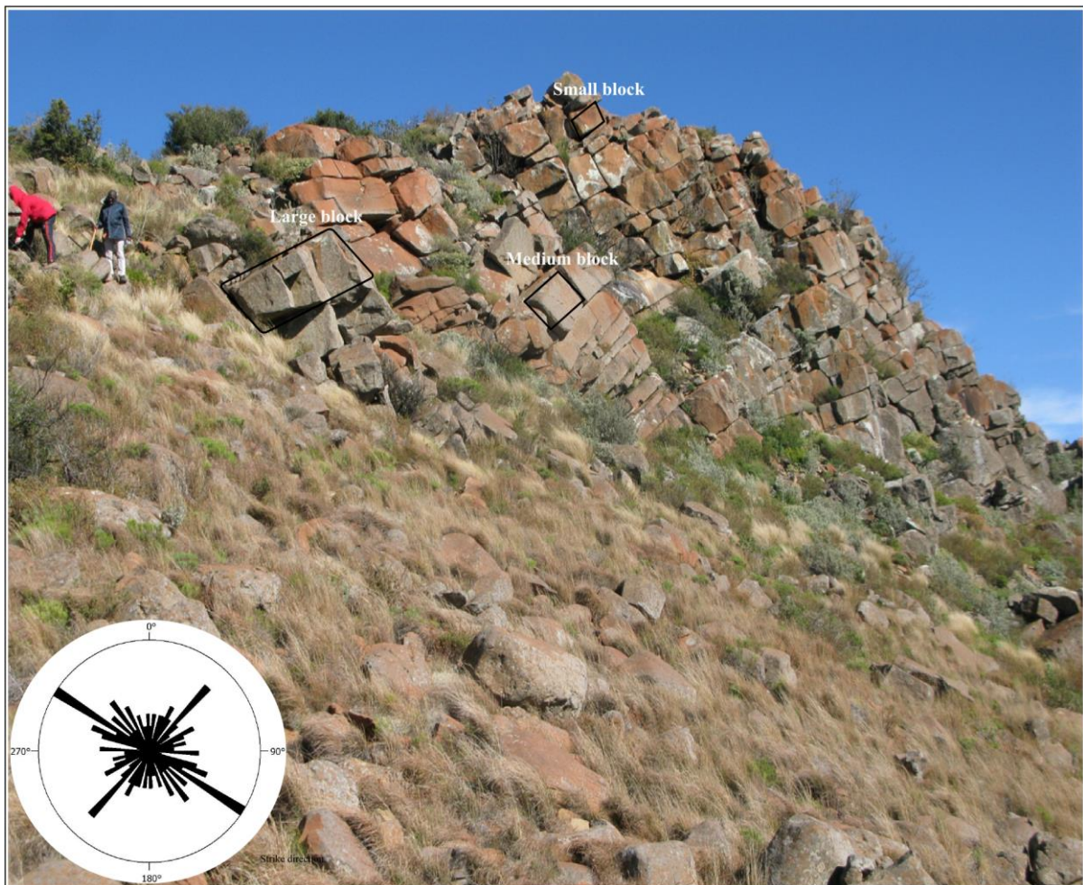
Figure 4.9: Photo of joints and blocks of dolerite sill from site 1 of GVS (Persons used as a scale \pm 1.70 \text{ m} ). The rose diagram on the bottom left shows strikes of 105 mapped joints from site 1.
