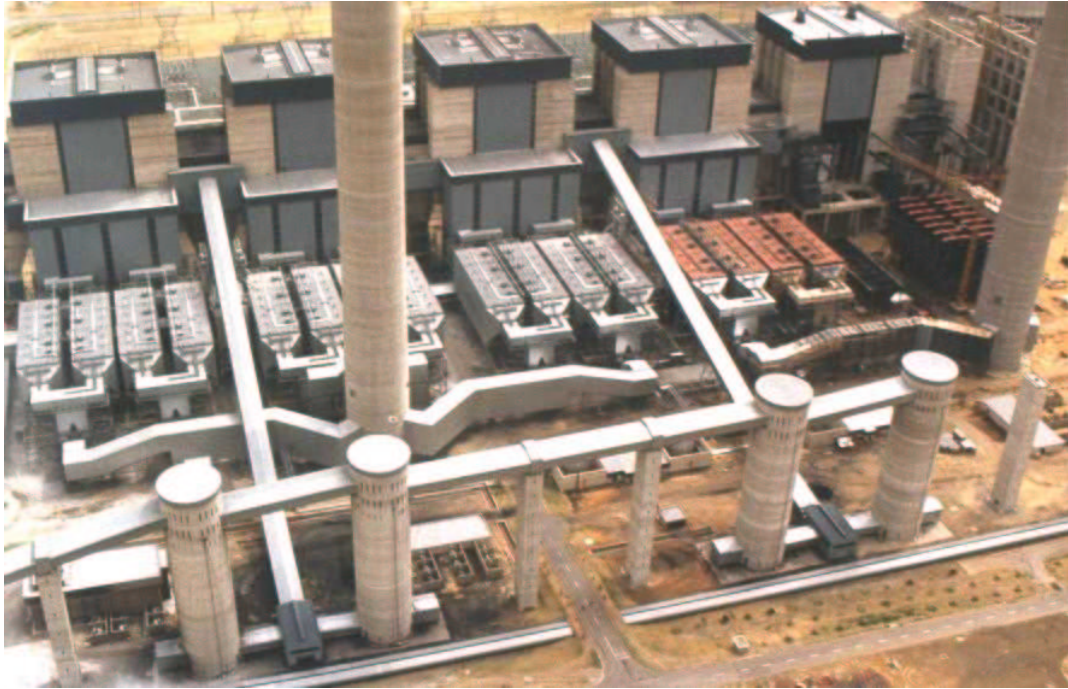
Plate 3.3 : Top view of Lethabo ESP Unit Casings
