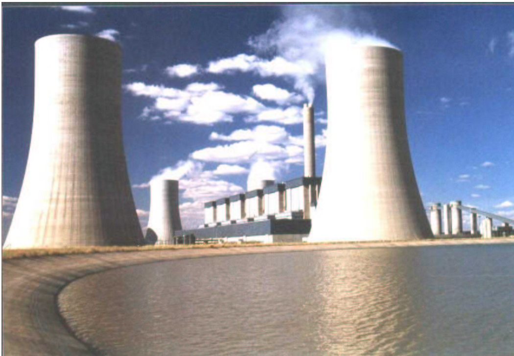
Plate 3.1 : Eskom's Lethabo Power Station
