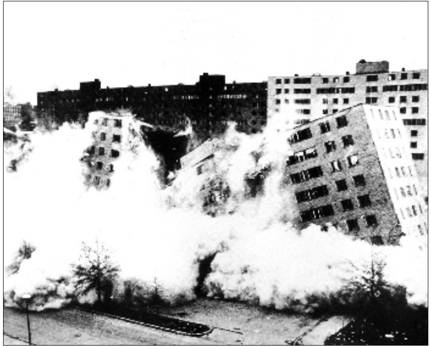
Figure 2. Minoru Yamaskai, Pruitt-Igoe Housing , St Louis, 1952-55 (demolished in 1972).
