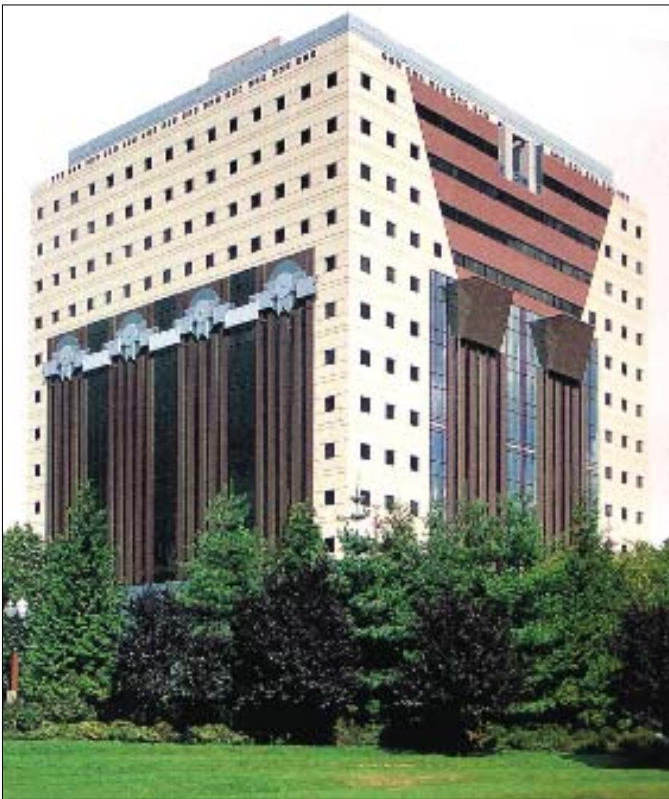
Figure 3. Michael Graves, Public Services Building , Portland, Oregon, 1980-1982.
