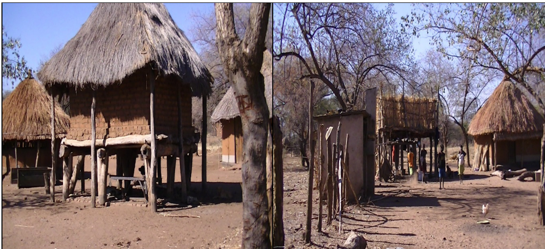
Plate 6.1 Defensive indigenous technology to withstand flood damage
