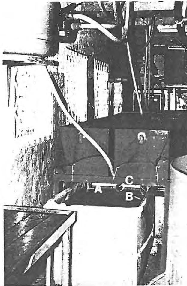
Figure 3a: Photograph showing sedimentation tank, with: A) water inflow pipe from culture tank, B) nylon stocking over inflow pipe (waste solid trap), C) outflow to biological filter.
