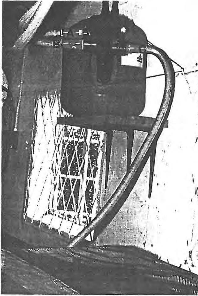
Figure 5a: Photograph showing activated carbon filter, with: A) inflow pipe, B) outflow pipe, C) backflush pipe.
