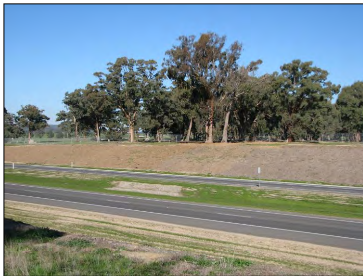
Figure 5.9: A photograph showing a dual-carriageway in Australia with raised roadside embankment either side of the road (van der Ree 2012).
