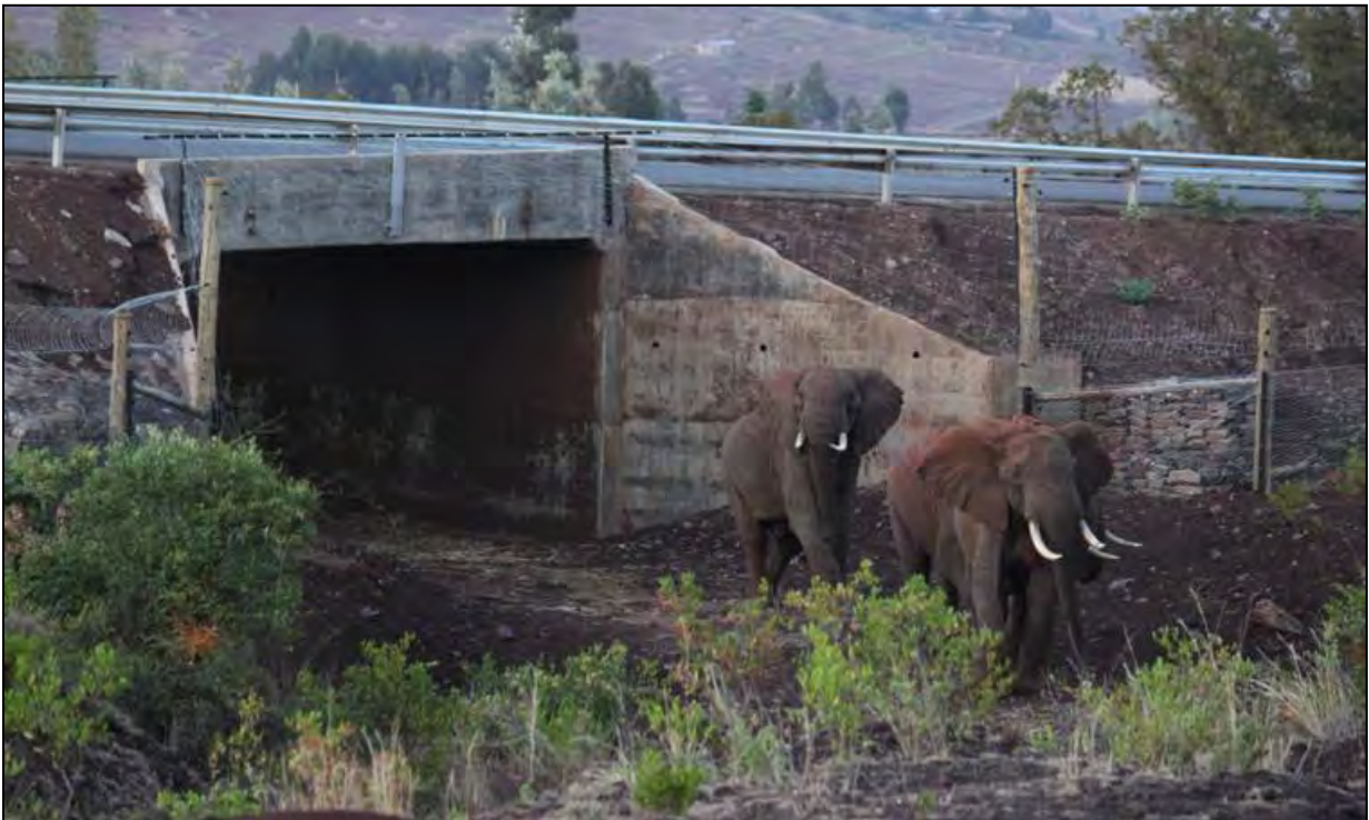
Figure 5.8: A photograph showing the Mount Elephant Corridor in Kenya with elephants utilising the underpass beneath the Nanyuki-Meru Highway (Mount Kenya Trust 2012). The underpass cost US$1 million to build.
