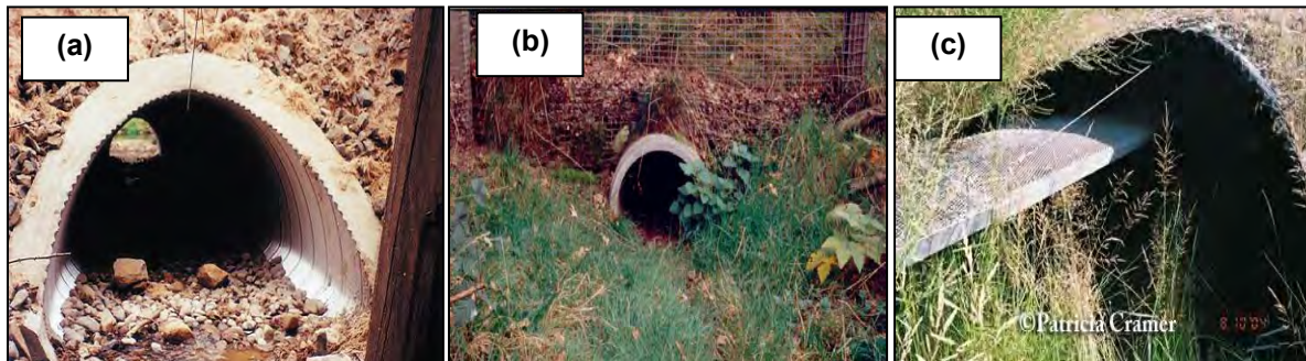
Figure 5.6: Three photographs showing different types of underpass design for small mammals, reptiles and amphibians (a) amphibian underpass using existing road features (FHWA 2012b), (b) fine mesh fence and culvert for small mammals in Europe (Evink 2002), (c) small mammal wooden plank crossing in a drainage culvert (Cramer 2004).
