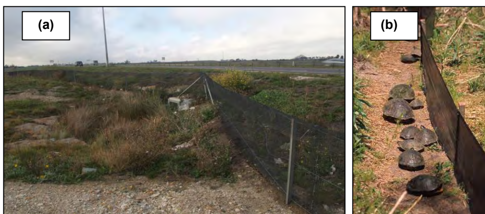
Figure 5.5: Two photographs showing how mesh fencing can be used to guide animals towards wildlife passages (a) small mammal wildlife passage leading to a culvert, Australia (van der Ree 2012), (b) Gopher Tortoise wildlife passage, Texas, USA (Lake Jackson Feasibility Study; Sewell 2004).
