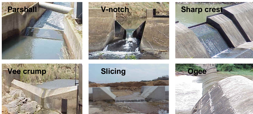
Figure 3.10 Types of flow gauging structures used by DWAF (website: http://www.dwaf.gov.co.za/hydrology downloaded in June 2008).
