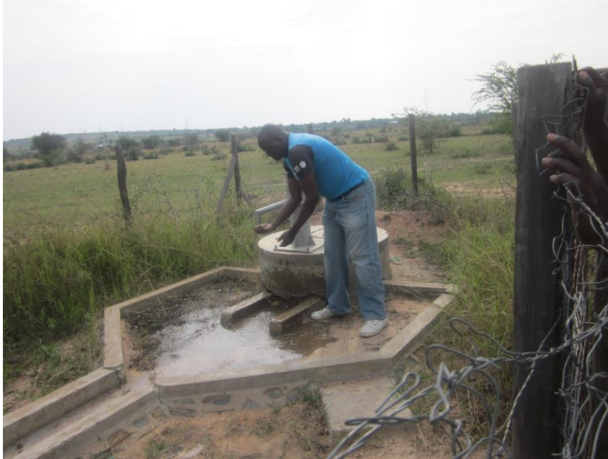
Figure 3.12 Abandoned improved source in Tito community.
