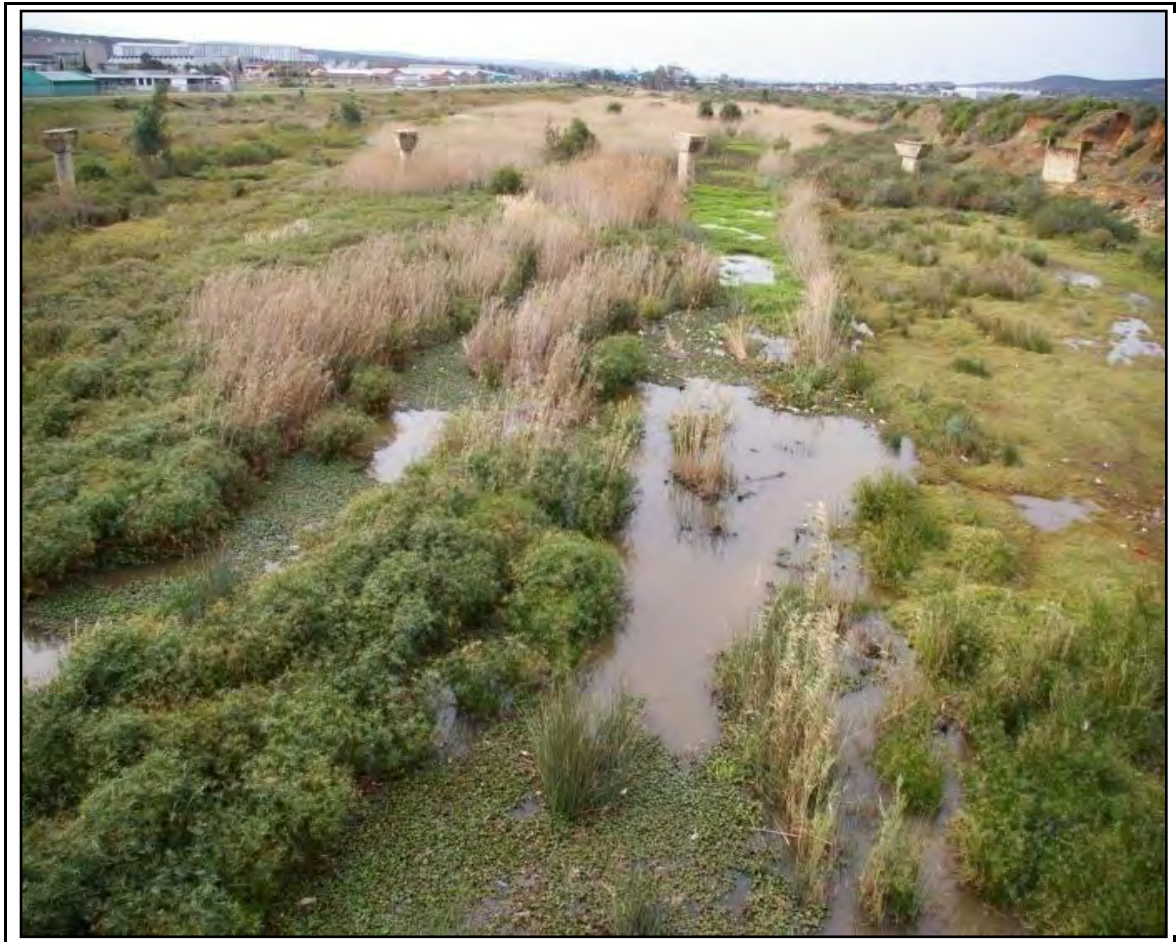
Figure 5.2: Spray zone (SZ) showing water hyacinth before spray and habitat degradation
