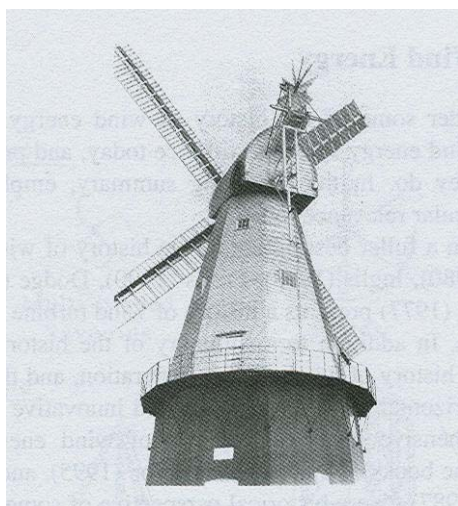
Figure 2.4 Horizontal axis lift type windmill 1
