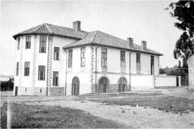
Figure 2. The new science block shortly after its completion in 1914. Zoology occupied the ground floor in 1916. Photograph from the Cory Library.
