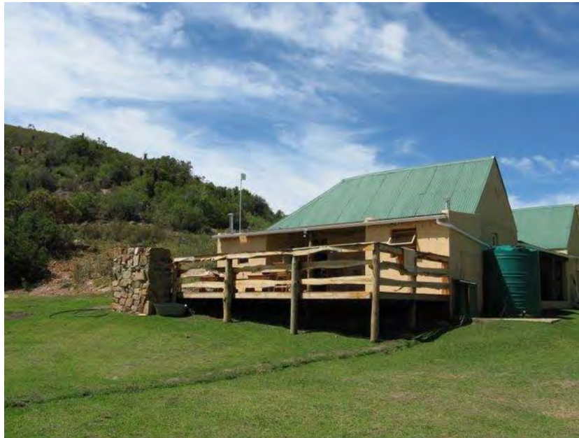
Figure 21. A view of the veranda. Photo taken January 2009.
