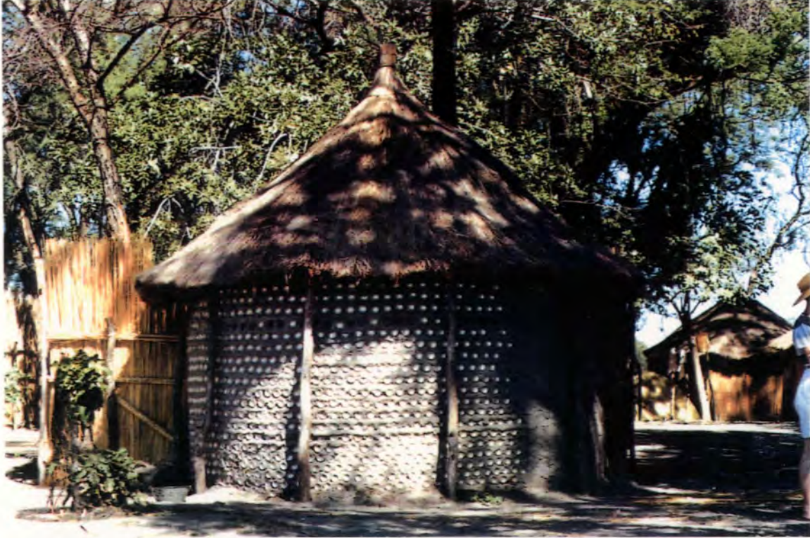
Empty cool drink and beer cans used in the construction of rural dwellings in Botswana. This is a practical use of waste materials but could not possibly be called Outsider Art.
