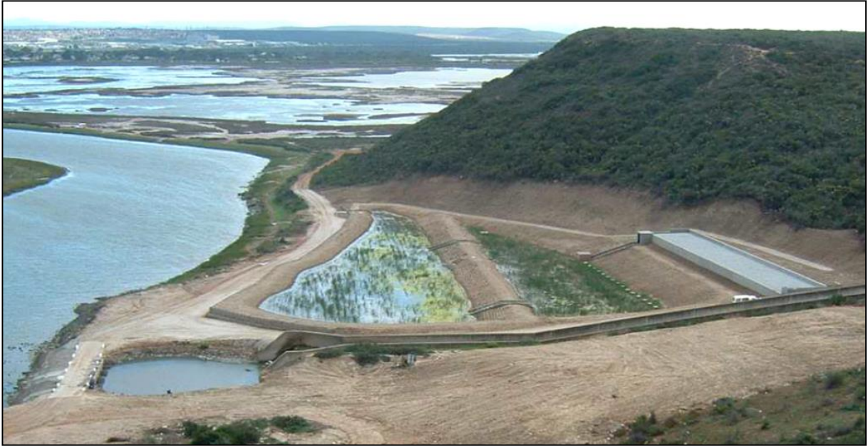
Figure 5: An aerial photograph of the Motherwell artificial wetland taken after completion in 2009. The wetland includes a primary reinforced concrete containment cell (right) and two secondary reedbed cells for treatment (SRK Consulting (Pty) Ltd, 2010).
