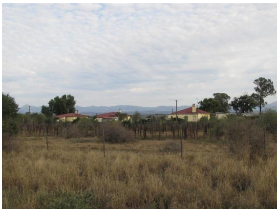
Figure 6.2: Transnet railway houses (Glenconnor, 2012)
