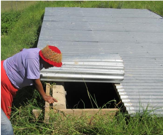
Figure 5.17: Nothemba demonstrates how difficult it is for her to get water out of her rainwater reservoir as it is so deep (Cata, 2012)
