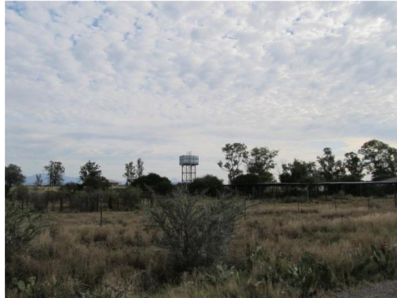
Figure 6.6: Glenconnor's town water tank (May, 2012)
