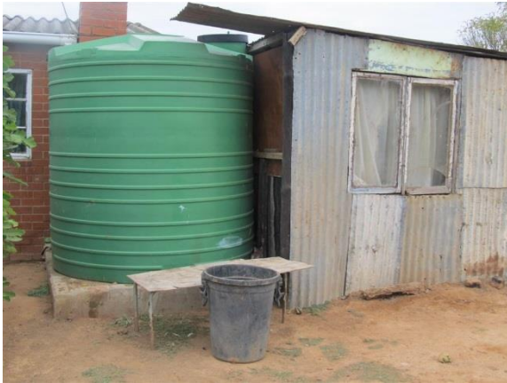
Figure 6.14: Mrs. Plaatjies’ rainwater tank adjacent to her kitchen (Glenconnor, 2012)
