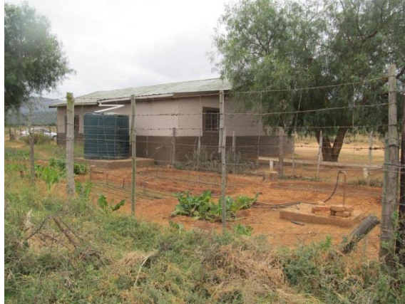
Figure 6.4: The primary school in Glenconnor with a vegetable garden and rainwater tank (2012)
