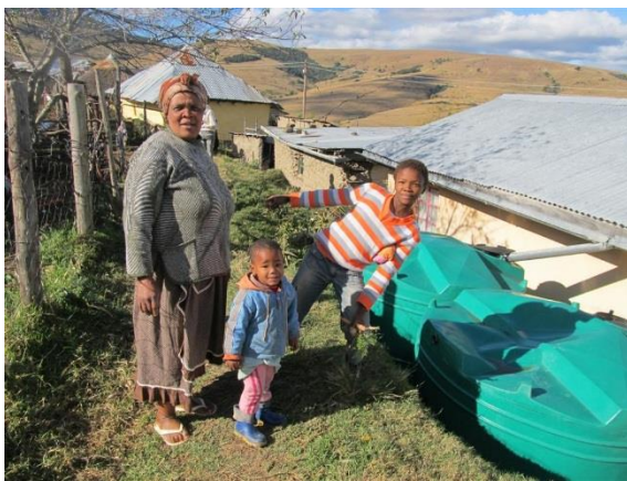
Figure 5.22: Bolekwa’s rainwater tanks at her house (Cata, 2013)
