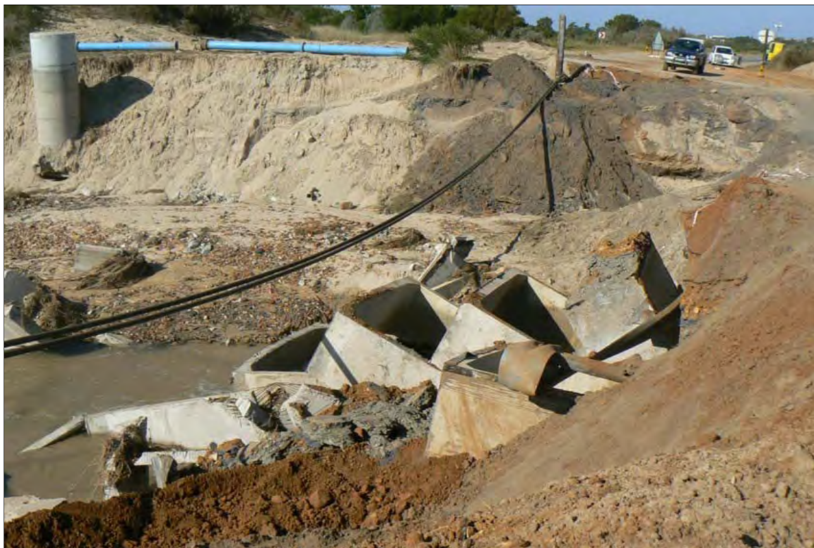
Figure 6-5: Remains of the former bridge across the Sand River following flooding along the Sand River in July 2011.
