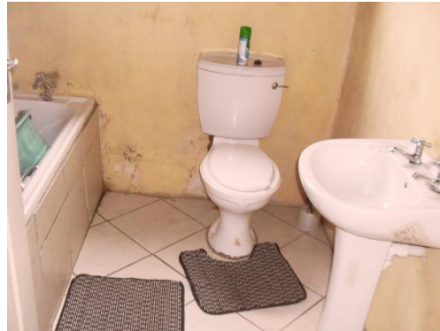
Figure 35 A recently installed indoor bathroom
