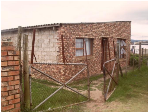
Figure 10 A house with incomplete improvements to the front
