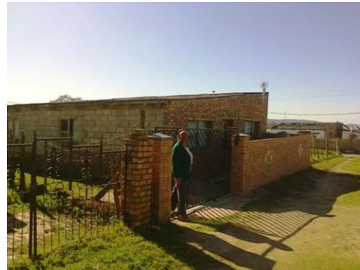
Figure 11 The same house two years later with security improvements
