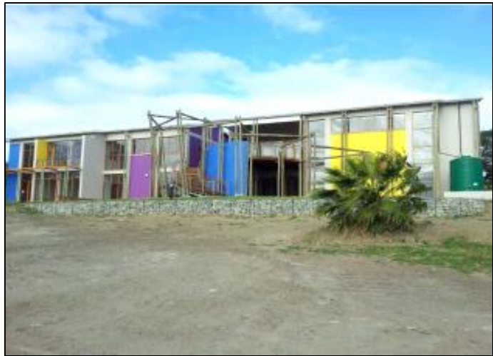
Fig 4.93: Building built to Keiskamma Art Project specifications, by ASPIRE source F. Danais.
