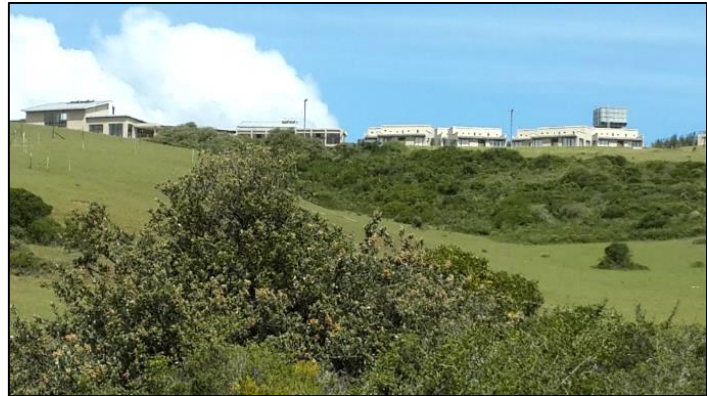
Fig 4.92: The Emthonjeni Project buildings (2014), source H. Osner .
