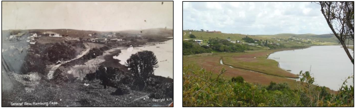
Fig 1.2: Photographs taken of the Keiskamma river, the postcard photograph on the left was taken in the 1930s, source C. Bailey, and the one on the right taken in 2014, source H. Osner.
