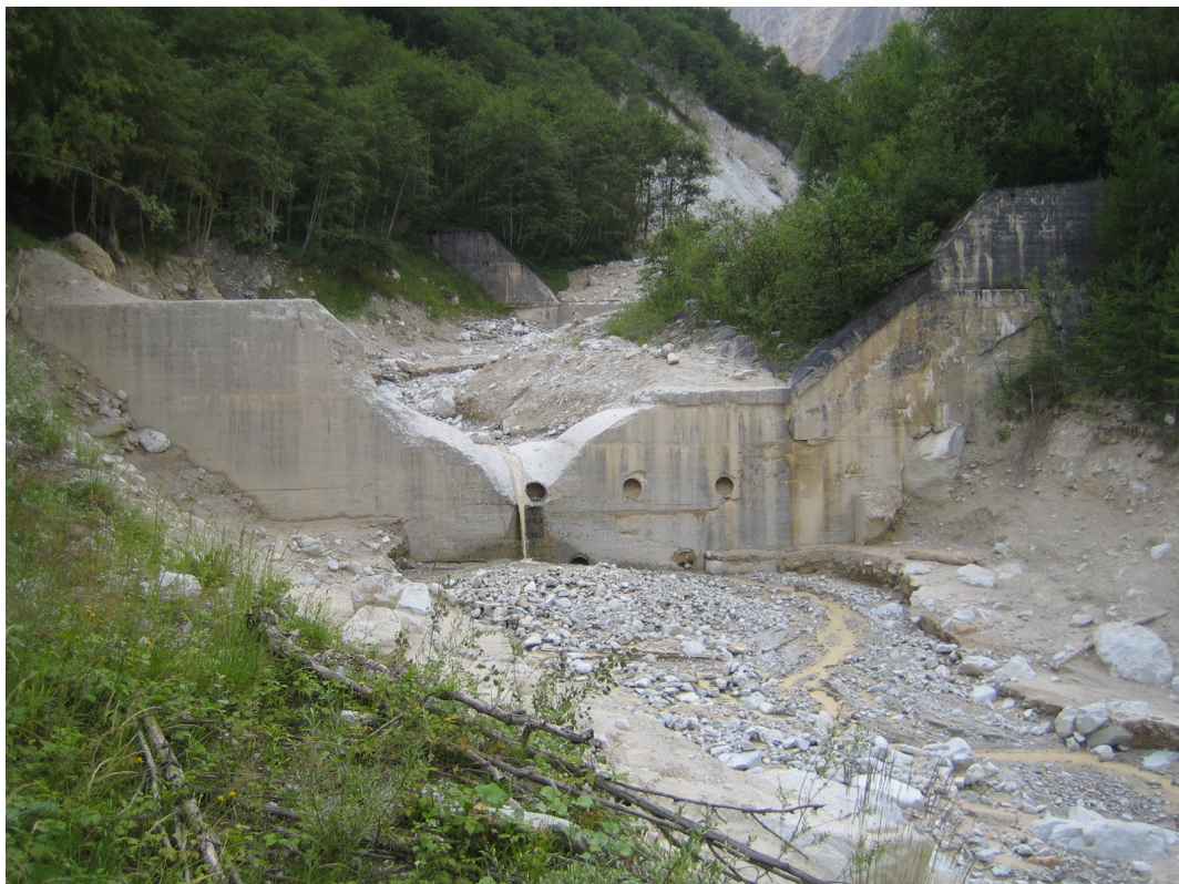
Figure A.8: Illgraben channel upstream of CD10 (Figure 4.1).
