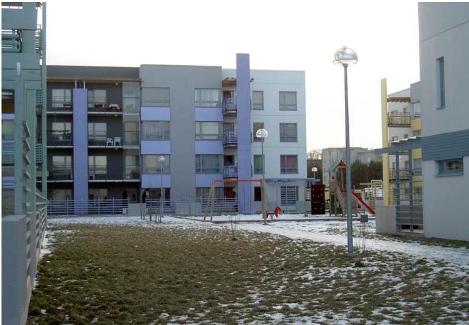
Figure 5. Example of a modern multifamily housing complex in Viimsi.
