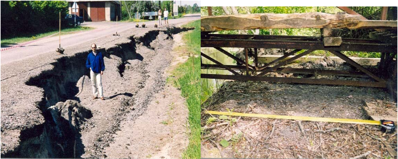
Photo 1. Fresh scarp of the Audru landslide and skidding tail of the bridge construction. Photos by Peeter Talviste, Pille Sedman.
