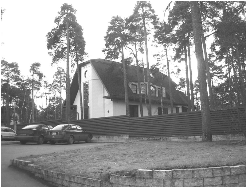
Figure 12. Nõmme, Tallinn (suburban low-rise housing area).
