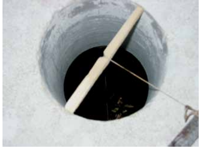
21 Centriranje položaja osovine mlinskog postrojenja (foto: Sanja Buble, 2008.) Centering the position of the axle of the mill mechanism (photo by Sanja Buble, 2008)
