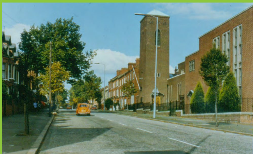
Figure 16: St Barnabas’s Church, Duncairn Gardens demolished to make way for a Business Park buffer zone.
