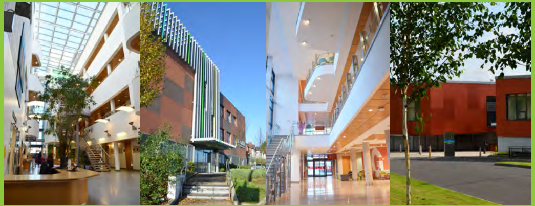
Figure 26 (right): Images of Wellbeing and Treatment Centres in Belfast – the focus on design quality has been well received and highly commended.
