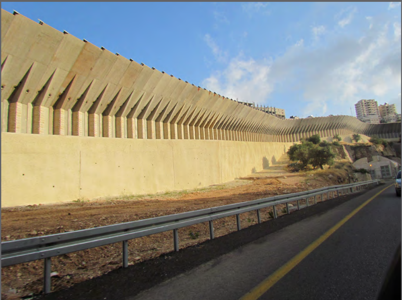
Figure 23: Motorway protected by a high security wall in Jerusalem.
