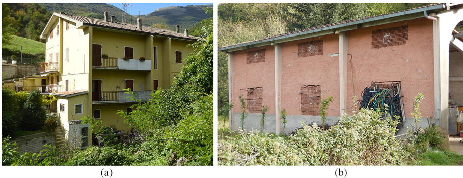
Fig. 16 a Building ID 41 in Arquata, Long. 42,46,33.64N Lat. 13,17,37.88E; b Building ID 5 in Grisciano (Accumoli municipality), Long. 42,43,51.57N Lat. 13,16,11.676E; Source EEFIT (2016)
