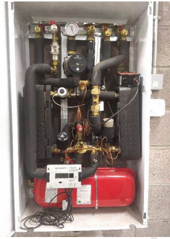
Figure 5: The dual heat exchanger sub-system
